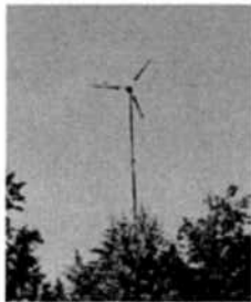
Guyed Monopole Tower
